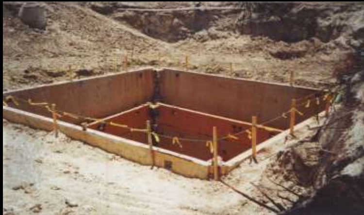
Trench Shields Connected at Corners
